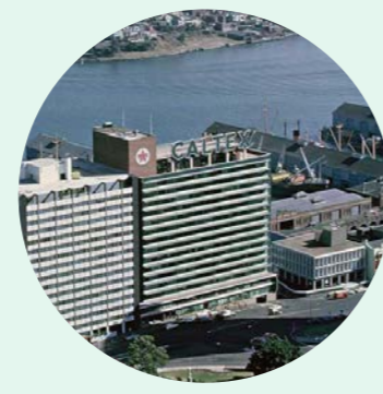
1957 Caltex House Australia's first all concrete skyscraper and the tallest building
